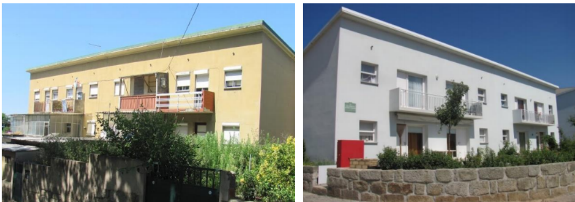
Figure 2. Image of the building before and after the intervention.
